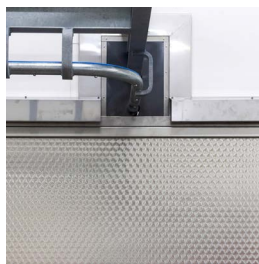
Rail passage with interrupted guide rail
