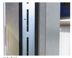
**Light Grid**Smart safety system is integrated into the side frames and eliminates contact with objects and people in doorway.
